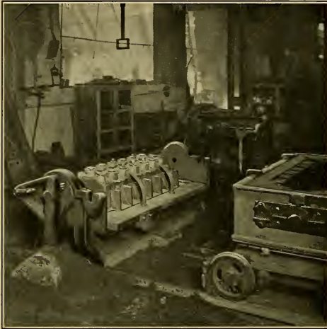
Fig. 58. Pattern Mounted on Roll-Over Jolt Machine.
